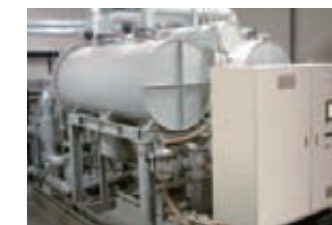
Adsorption Chiller Fiscal 2005 to 2007 New Energy and Industrial Technology Development Organization (NEDO) New Solar Energy Systems Technology Development Project Photo: MAYEKAWA MFG. CO., LTD.
